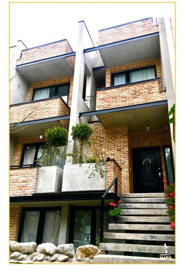
The 50 years old house rebuild by some materials that remained during the destruction process and reused in the facade as brick and stones.
